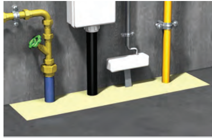
Mix service penetrations
